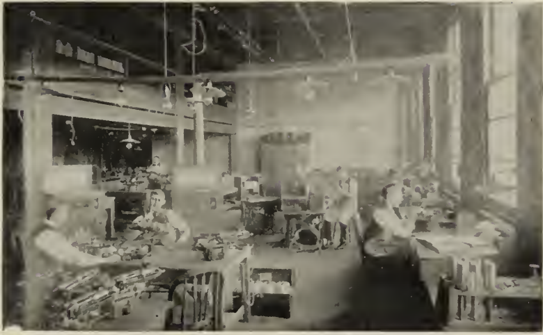
Assembling and Testing Department—Edison Phonograph Works.
